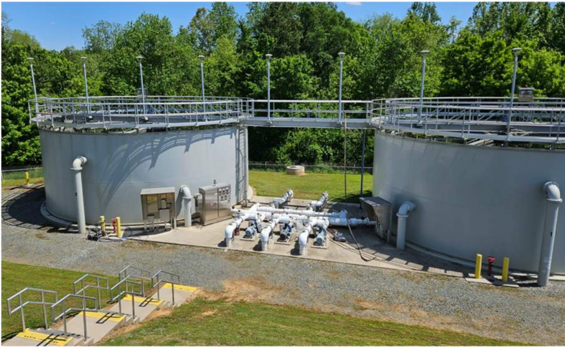
Figure 8. RAS pumping station between secondary clarifiers.
