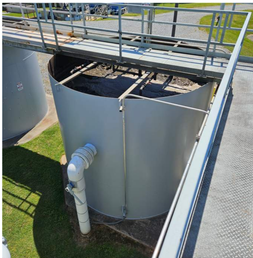
Figure 13. Sludge holding tank number 2.
