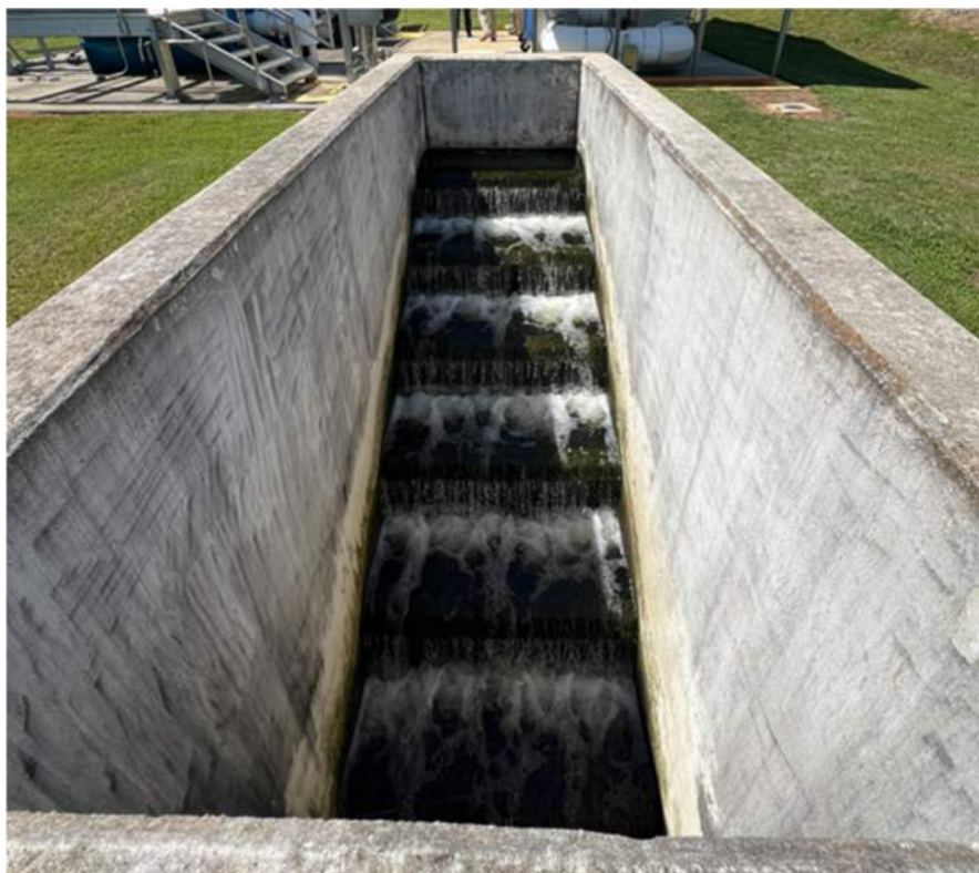
Figure 11. Cascade Aerator.
