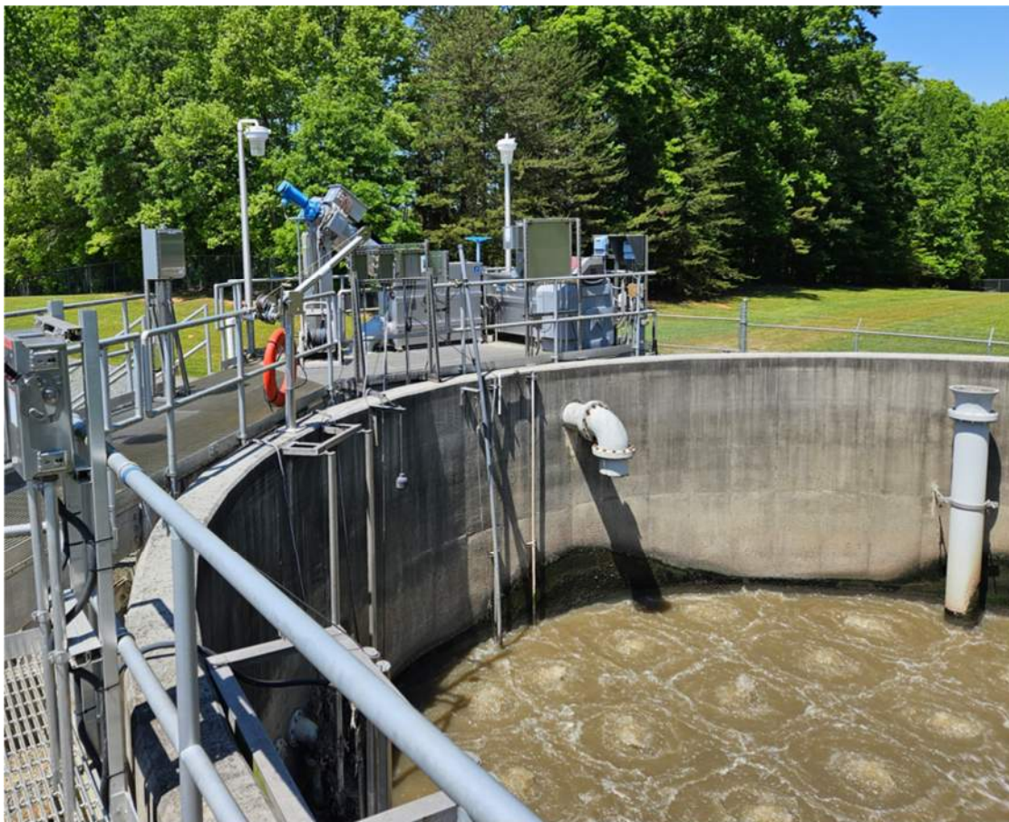
Figure 4. Equalization basin.
