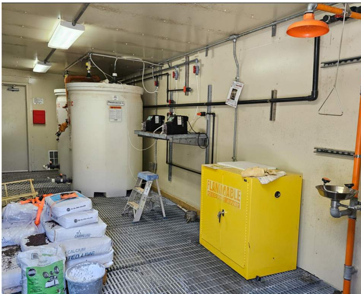
Figure 5. Chemical storage room showing metering pumps and old (abandoned) day tanks. Larger 6,600-gallon storage tank is located outside this building.
