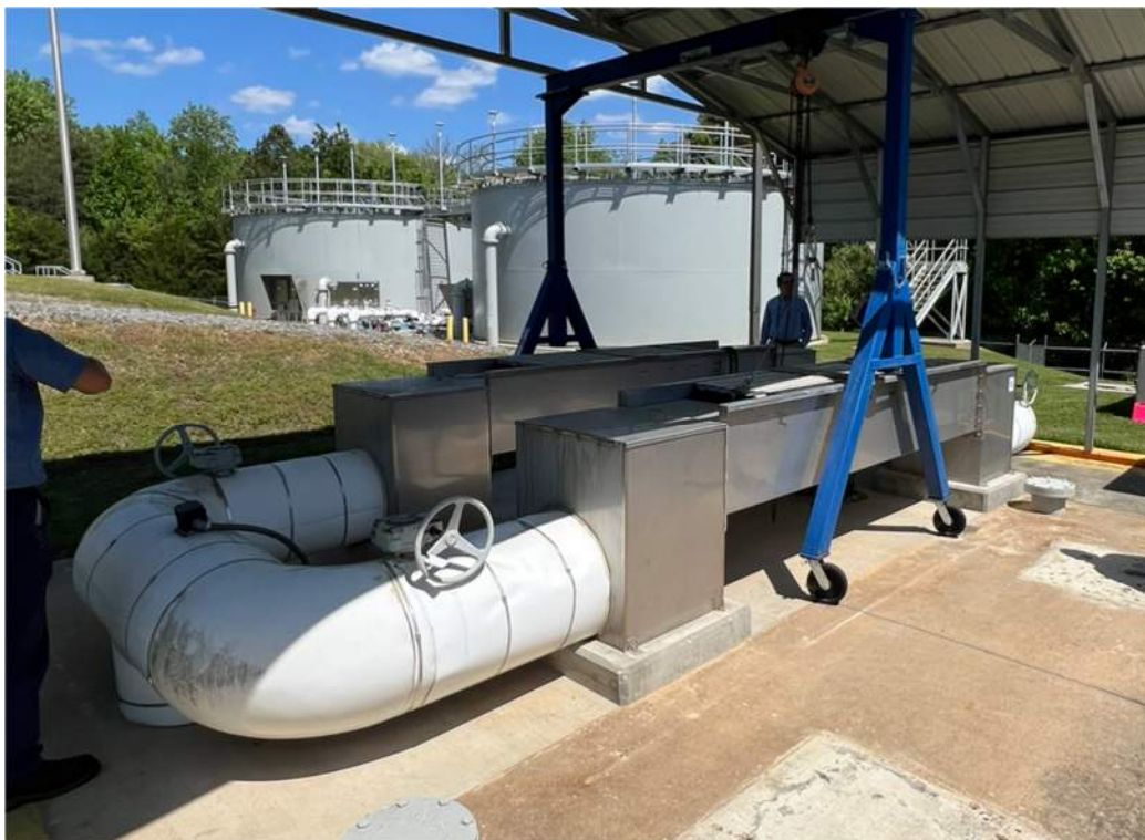
Figure 10. UV disinfection facility.
