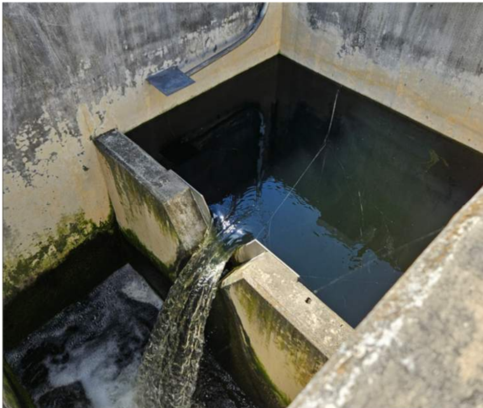
Figure 12. V-notch weir inside effluent monitoring box.
